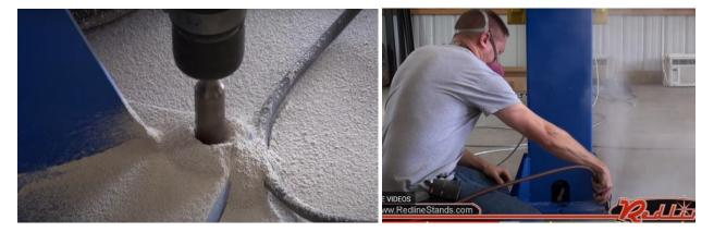
In this step, we discuss the optional use of adhesives to help the anchors secure to the concrete. If you do not wish to use an adhesive, you can skip this step. However, we recommend this step as it will help to ensure your concrete anchors do not loosen over time.
