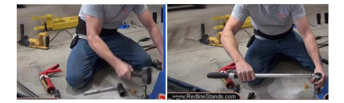
Now that the first tower is secured to the concrete, we'll wait the recommended amount of time for the adhesive to cure as per the chart on the tube, and then we'll install the shims that come with the lift to get the tower plumb. You'll use a level against the side of the tower, loosen the freshly tightened anchor bolts, and then add shims as needed until the tower is perfectly plumb, and then retorque the anchors.
